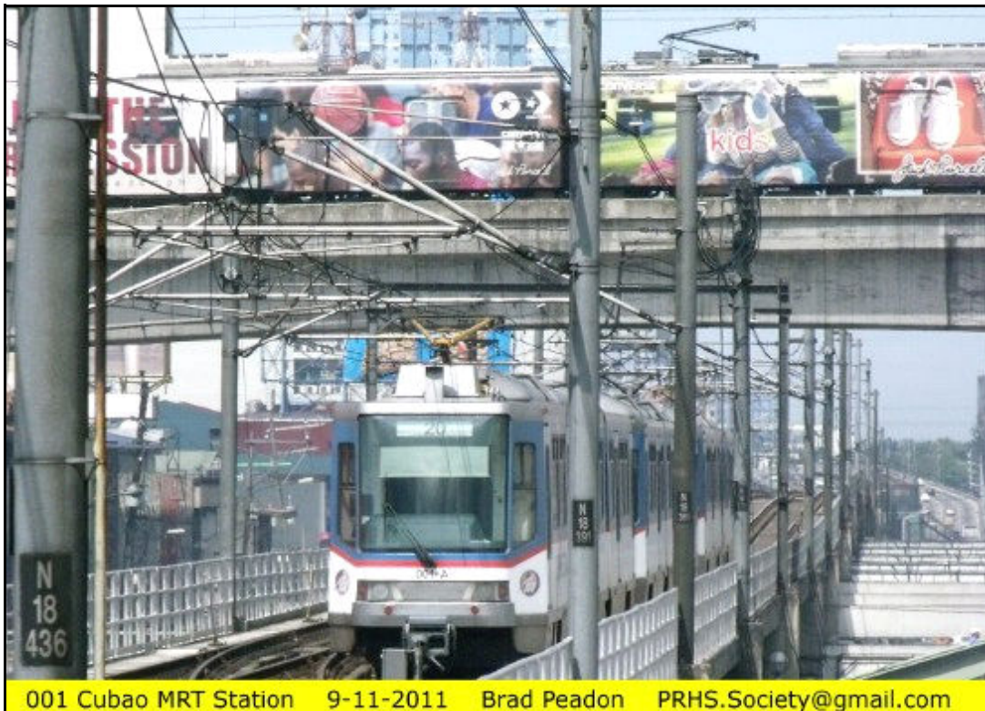
LRT2 passing over the top of the MRT3 system at Cubao.
